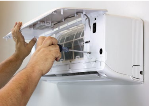
Back out electrical panel screws
