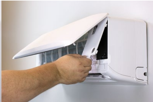
Remove electrical access panels [2]
